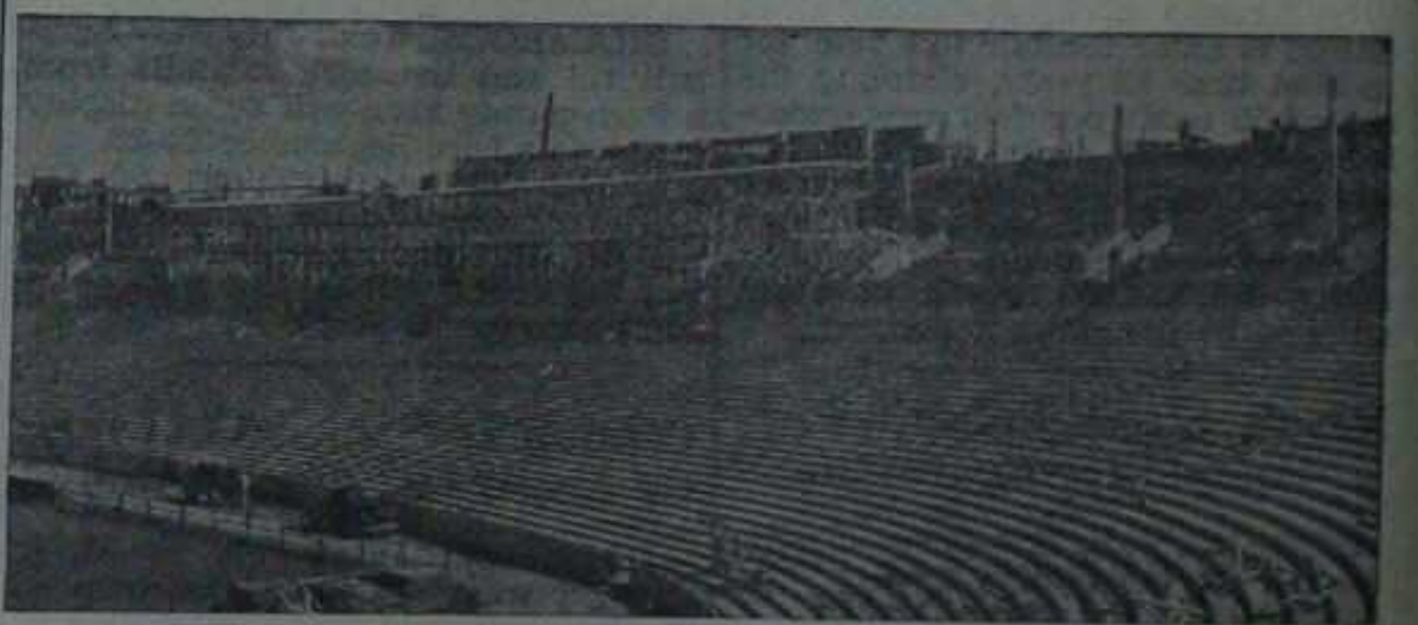
THE COTTON BOWL at the State Fair of Texas, Dallas, as it will appear when completed is shown in the photo at top. Lower shot shows the progress made on the project to date. When completed the new Cotton Bowl will have a seating capacity of 67,435 as against the former Bowl's capacity of 45,195.
