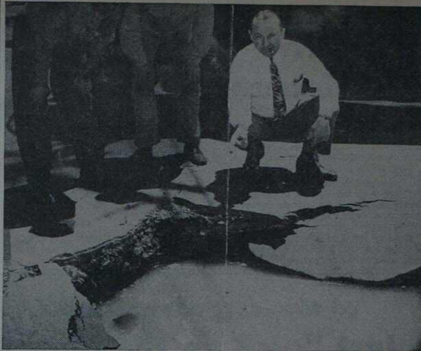
HERB WEDEWEN, REGIONAL SALES MANAGER for Rock-Ola in Erie, Pa., points out the spot where his car broke thru the street as he was returning home after a swing thru his territory. A sewer, backing up, weakened the pavement, causing the break-thru.
