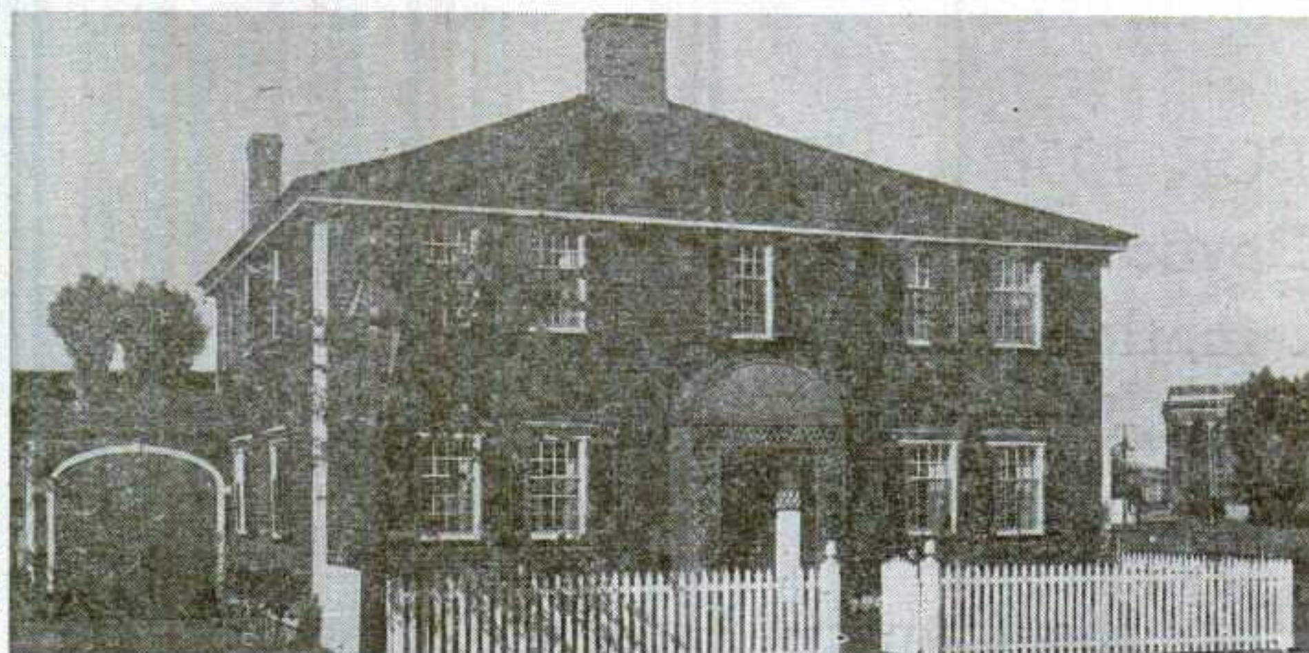
The Gilbert house is a typical farm homestead of its day. Originally erected in West Brookfield, Mass., in 1794, its hand-hewn timbers in some cases are 30 feet long, assembled with wooden pegs and hand wrought nails.
