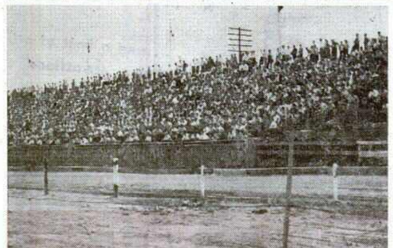
Low-cost bleacher-type stand at the Shelby, N. C., Fair was built on man-made hill, graded step-like to permit easy setting of seats. Upper photo shows almost full length of the 3,500-capacity stand; lower one gives close-up of native-stone retaining wall.
