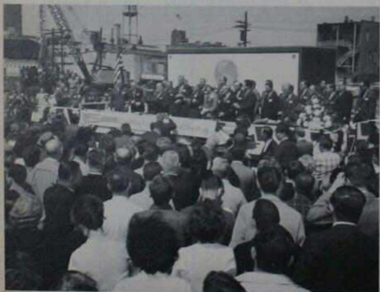
CHICAGO'S MAYOR RICHARD J. DALEY receives a standing ovation as he mounts the rostrum to congratulate Seeburg executives and employees for helping the city's urban development program by constructing a giant $15,000,000 manufacturing complex adjacent to the present Seeburg plant. Daley and Delbert Coleman, Seeburg board chairman, turned the first shovel of earth last Thursday (10) morning and work began immediately afterward.
