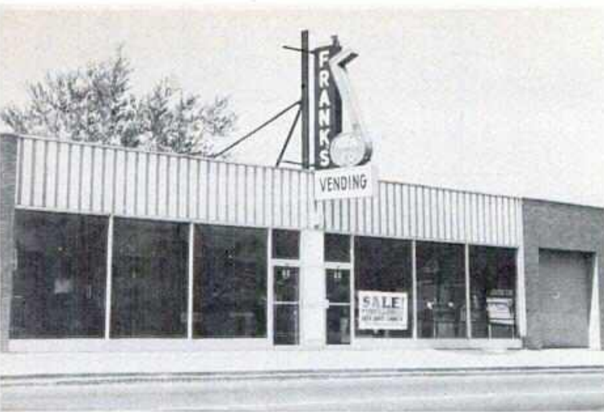
NEW HOME OF FRANK'S MUSIC CO., Detroit, is this spacious, modern building at 60 West Eight Mile Road. The new structure offers 8,100 square feet for one of the area's largest music, games and vending operations.
