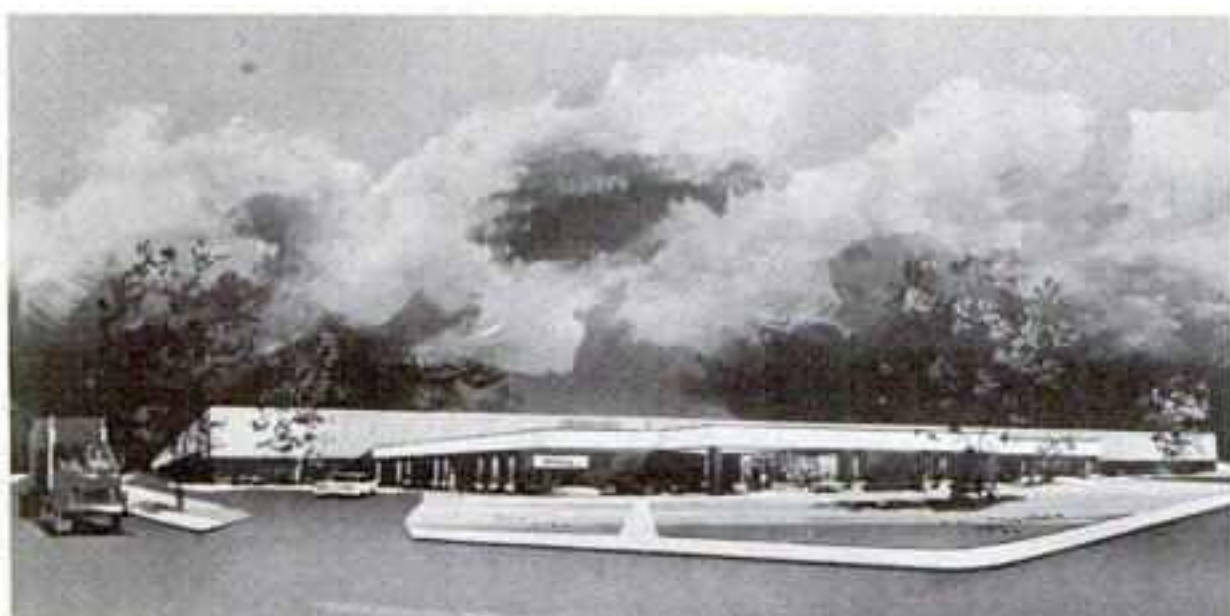
NEW HEADQUARTERS for the Wico Corp. in Nilus, Ill., will be ready in early 1971. The building, still under construction, will replace old offices and plant and provide 250 percent greater floor space.
