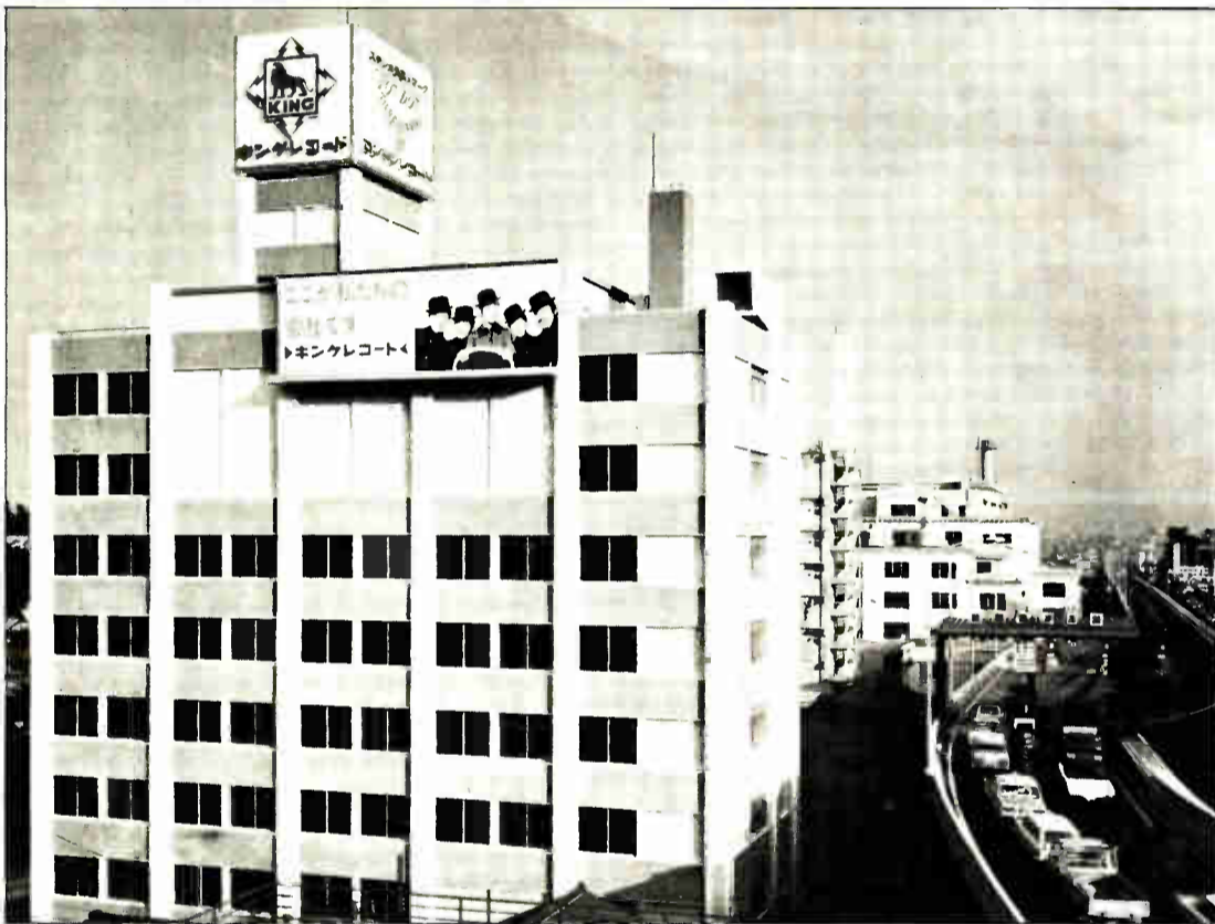
▲HEAD OFFICE housing EXECUTIVE SUITES, RECORDING STUDIOS AND OTHER FUNCTIONS WITH APPR. 300 PEOPLE.
