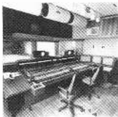
1987. STUDIO 2—DISCRETE CUSTOM CONSOLE, 32X12X24, WITH NECAM I.
