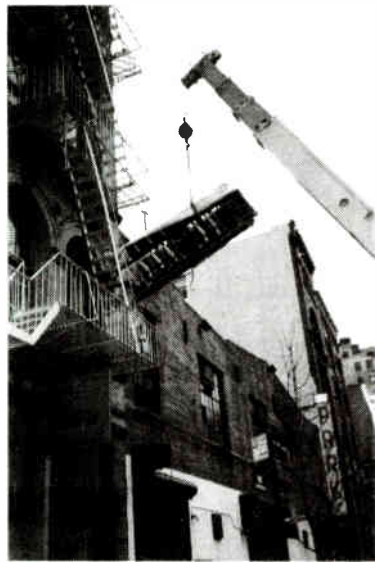
Kampo Cultural Center Studio takes delivery of an SSL 4056G console through a second-floor window—the only way it would fit.
