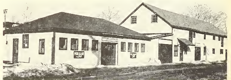
Nyack Slate's new manufacturing, distributing and operating facilities.
