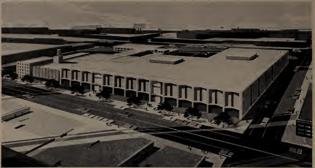
Seeburg’s plant at 1500 North Dayton Street. Housing two thousand employees, measuring more than 360,000 square feet, its construction was a joint project of the corporation and Chicago’s Economic and Cultural Development Committee.
