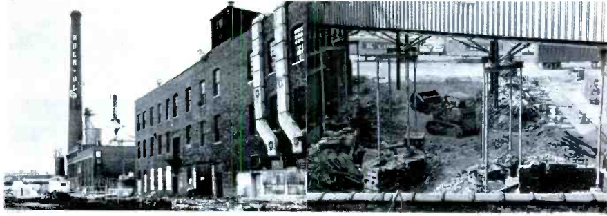
Work progresses on Rock-Ola factory "facelift"
