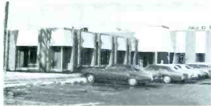
A view of the front of the building which appears to be undamaged. It was reported, however, that some automobiles and the Midway sign were damaged.
