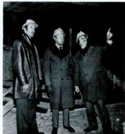
Pictured inside the soon-to-be-completed Marriot Hotel are (l-r): Don MacLagen, sales manager of the Holiday Inn Mart; Granger; and Marriot sales manager Michael Campa.
