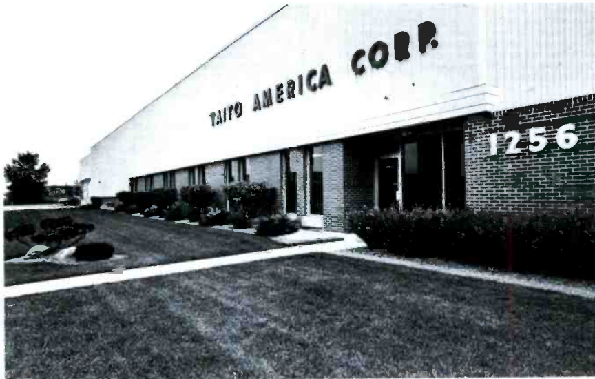
NEW HEADQUARTERS — Taito America's new corporate headquarters in Elk Grove Village, Ill. is a 60,000 square foot facility housing a modern factory and full administrative offices. "Qix," the first game to be produced in the new facility, began rolling off the assembly lines in September.
