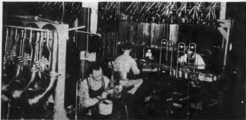
Assembly-line production at Conn's, with standardized parts, speeds output, facilitates repair work: is now restoring to pre-war levels supply of trumpets, trombones, tubas, larger-bore French horns, bassoons and oboes.
