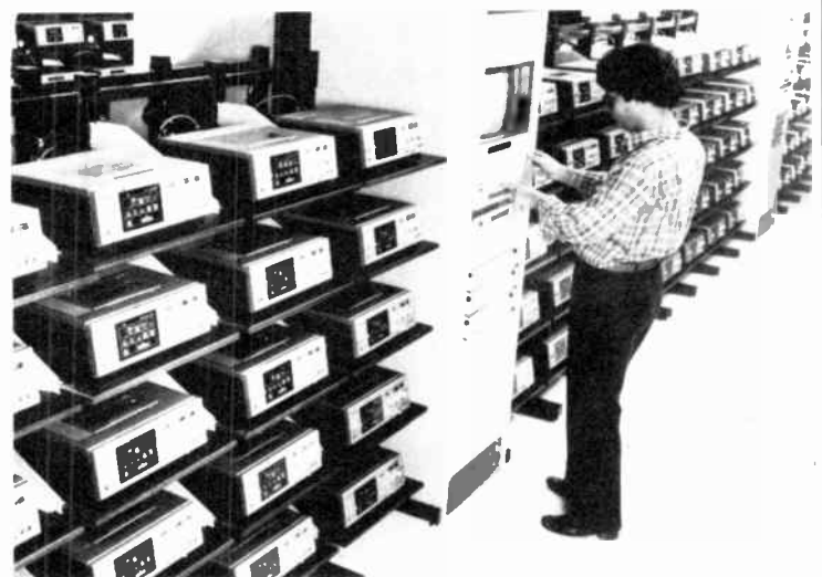
Capacity of Vidtronics new facility will be over 7 million cassettes a year
