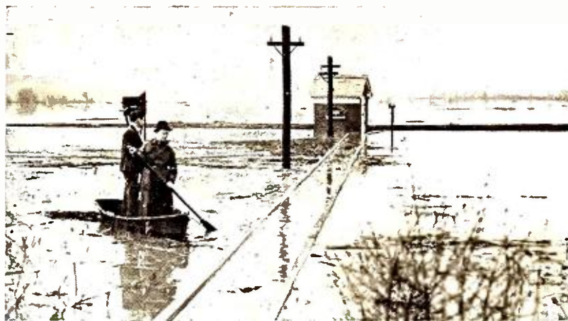
A FEW MORE INCHES —And the dog house of WJSV, CBS Washington station, would have been in the Potomac. Water rose almost to the tuning inductances. Just a bit more and WJSV would have been without its transmitter, located on the Potomac near Alexandria.
