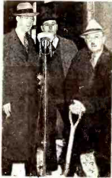
NEW STUDIOS —WCCO staged a special broadcast when work was started on its new studios, to be ready next March. Welding shovel and syllable are, left to right, C. R. Jacobs, CBS manager of construction; Hugh S. McCartney, WCCO chief engineer; Earl H. Gammons, WCCO general manager.
