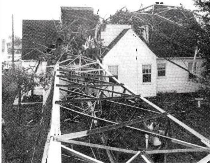
WHEN A TORNADO wrecked two towers of KMBC, Kansas City, Aug. 25, one of the towers, 544 feet high, fell on this house, 250 feet from the tower base. The antenna broke in the center before falling. Occupants of the house narrowly avoided injury [see story on page 42].
