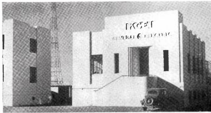
LAST WORD in modern design and construction is this new transmitter building, located at Belmont, Cal., of KGEI, General Electric international shortwave station in San Francisco. Operating with 50,000 watts, the station broadcasts on 6190, 9530, 15330, 9670 kc.
