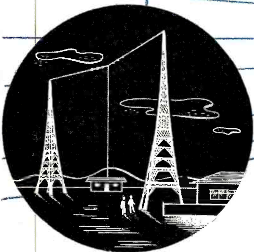
1934 One of the first directional antenna arrays for broadcasting. Designed for WOR to concentrate signals in service area, eliminate radiation over ocean.
