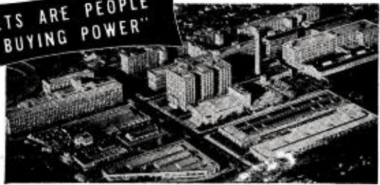
Air View, National Cash Register Co. Plant, Dayton, Ohio.
