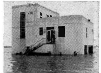
WWL's flooded transmitter
