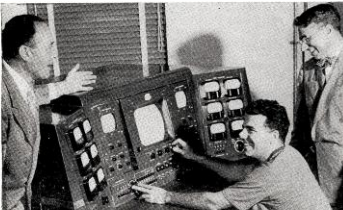
ENGINEERING phase of the WNHC-TV operation is discussed by Manager James T. Milne (l), Chief Engineer Vincent DeLaurentis (center) and Aldo DeDominicis, promotion manager. Until lines are installed from studios to transmitter the video portion of WNHC-TV programs from DuMont network is received via relay at transmitter. Audio line terminates at studios. All slides and films are handled at transmitter.
