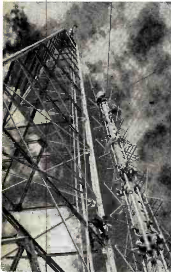
SUPER turnstile for KECA-TV Los Angeles is raised to top of the 303-foot supporting structure. Tower for the ABC video station is on crest of Mt. Wilson, 5,999 above sea level.
