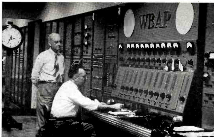
A FLIP of the switch by Engineer Roy Bond (seated)—and WBAP Fort Worth's complete new AM studios went into operation June 18. Standing by is R. C. Stinson, WBAP director of engineering. The 40-ft. control panel in front of Mr. Bond is part of the new RCA custom-built equipment installed in the new radio-television center in Fort Worth.
