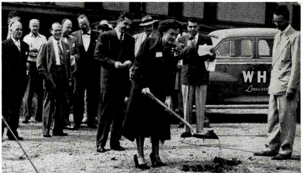
A REPRESENTATIVE WHAS Louisville listener, Mrs. Paul Eubank, moves the first shovel of earth for erection of the station's television tower. Immediately in back of ville's Mayor Charles Farnsley, in black bow string tie. Holding the portable microphone is Master of Ceremonies Pete French. Technical Director Orrin W. Towner is at Mrs. Eubank is Victor Sholis, WHAS director, and Louis- far right.
