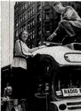
MODEL Helen Pastorius helps Manager Charles E. Dewey Jr. of WKJF (FM) check antenna before inaugural of station's Transitcasting service on city's busses. Holding the ladder is C. F. Kreitzer, WKJF commercial manager.
