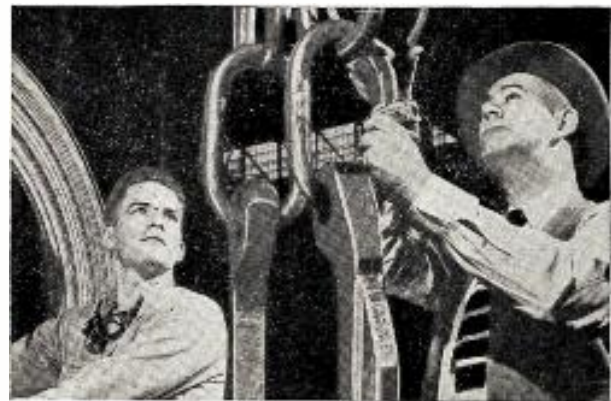
5. Here a supervisor is making a periodic check with calipers on the chains and coil hooks of John's conveyor. Evidence of defects or over-strain means prompt replacement to prevent accidents.
