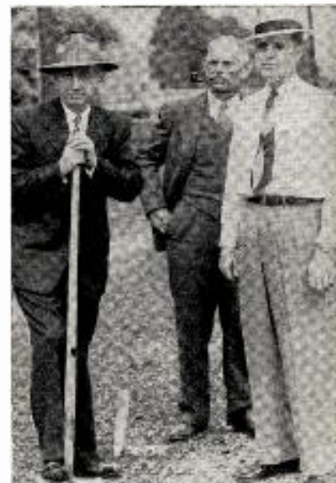
GROUND is broken in Memorial Day ceremonies at the site where WTVR (TV) Richmond will build new TV facilities. Wielding the shovel is Wilbur M. Havens (l), owner of the station, as Harry Jordan, contractor, and James W. Kyle (r), WTVR chief engineer, stand by. WTVR, in its third year of operation, expects to have its modern studios ready for programming in the fall.
