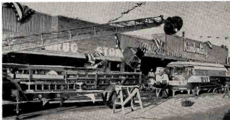
WKY-TV's high-flying parabola goes up on the end of an Oklahoma City Fire Dept. ladder truck.
