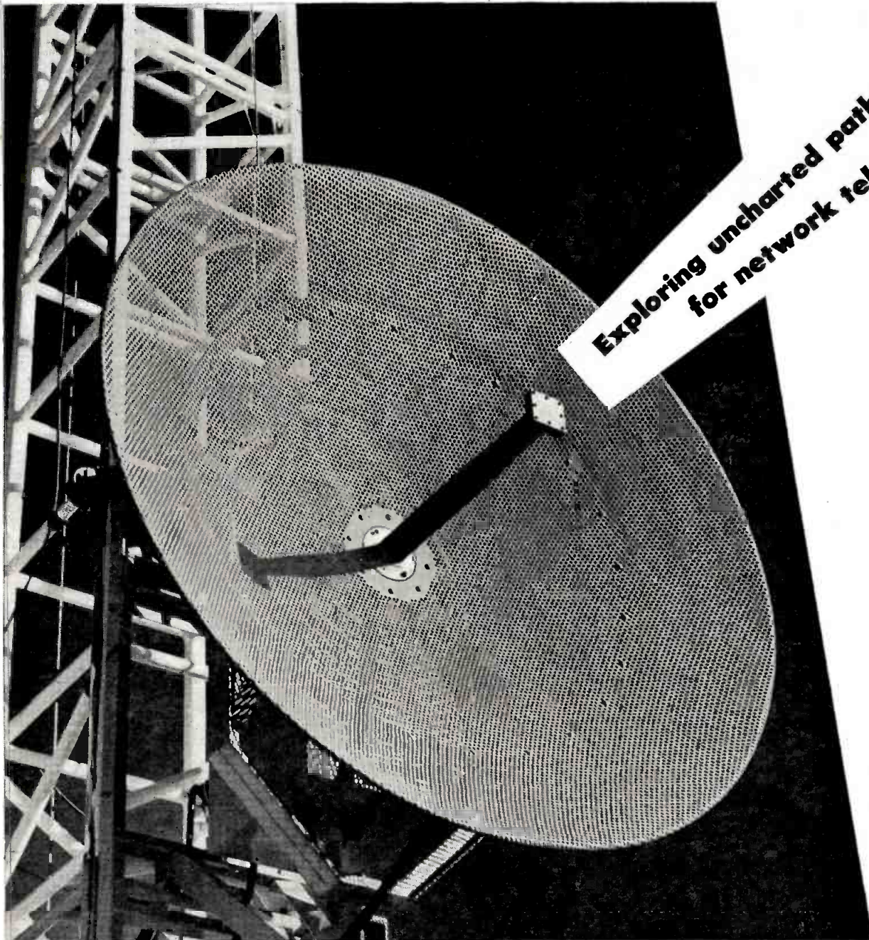
Portable microwave reflector—used in locating best radio relay routes
