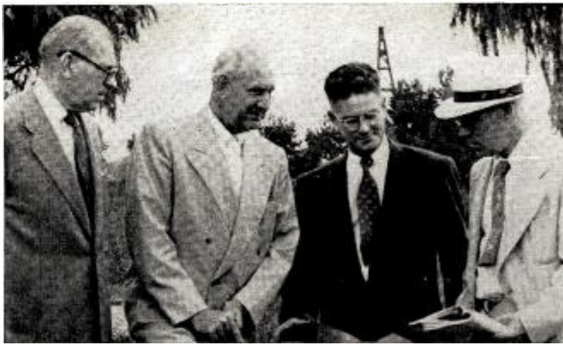
WCAM Camden, N. J., on Aug. 25 began construction of its new transmitter site at Pyne Point Park in Camden. On hand were (l to r) Herbert L. Wilson of Herbert L. Wilson Assoc. Engineers, Washington, D. C.; Mayor George E. Brunner of Camden; John Cleary, WCAM manager, and Willard C. Schriver, station director.
