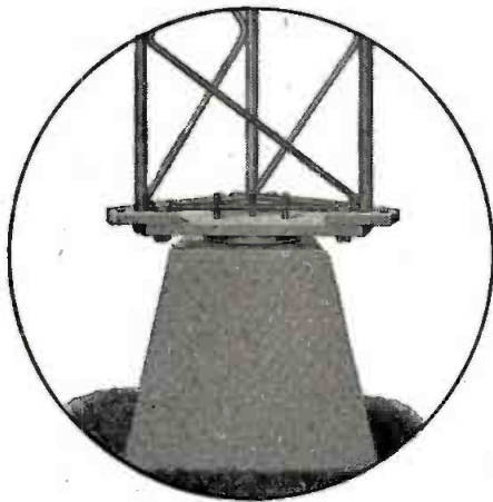
Typical central pier arrangement for non-insulated tower. Other arrangements are possible to meet specific conditions.
