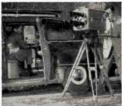
Compact GPL studio camera chain fits easily in station wagon, and may be operated from there, drawing power by cable from studio and returning signal to transmitter.
