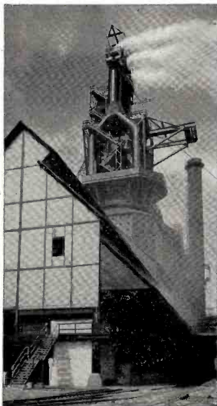
Furnace "J", the seventh blast furnace at Lackawanna Plant, is over 105 feet high. Its construction took 6500 tons of steel plates, shapes and castings. A turbo-blower supplies the 100,000 cubic feet of air per minute needed for the blast.
