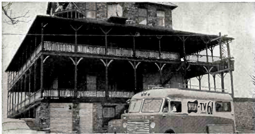
WHUM-TV studio building is shown above. From here signals are beamed via microwave to their transmitter site 22 miles north of Reading, Pa.
