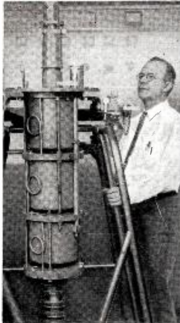
Kenneth Cooke, Chief Engineer, (photo left) stands alongside a Klystron tube used to amplify the WGBI-TV signal to peak power before it is beamed from a G-E 12 KW transmitter (photo right).
