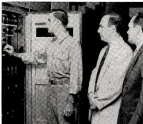
WDSU-TV New Orleans goes to 100 kw maximum power on Ch. 6 as engineer John Dickenson throws the switch. Edgar B. Stern Jr. (c), president of WDSU Broadcasting Corp., and Lindsey Riddle, station's chief engineer, are witnesses to the power boost ceremony.
