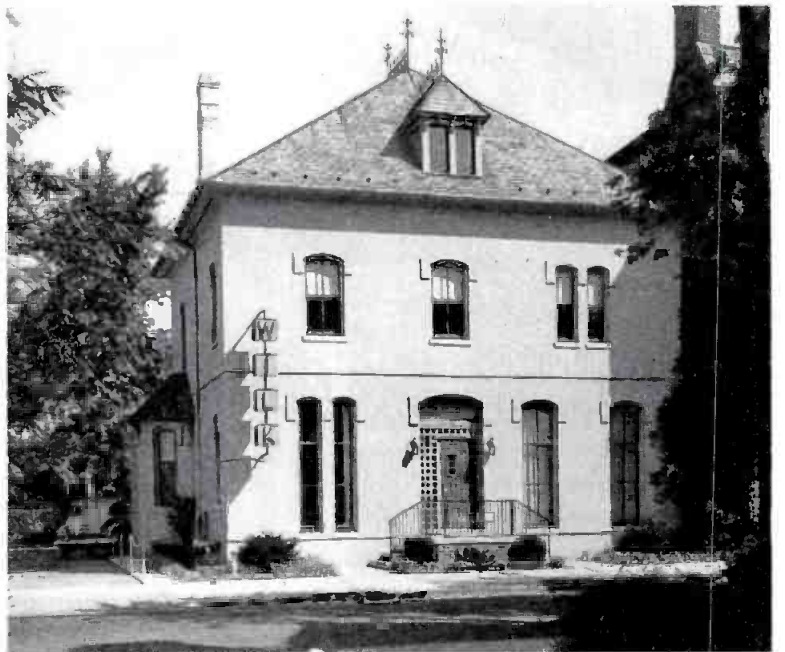
WILK-TV, Wilkes-Barre, Pa. This converted residence is the home of WILK. The antenna, a G-E Helical, is on Penobscot Mountain, elevation 2350 feet.
