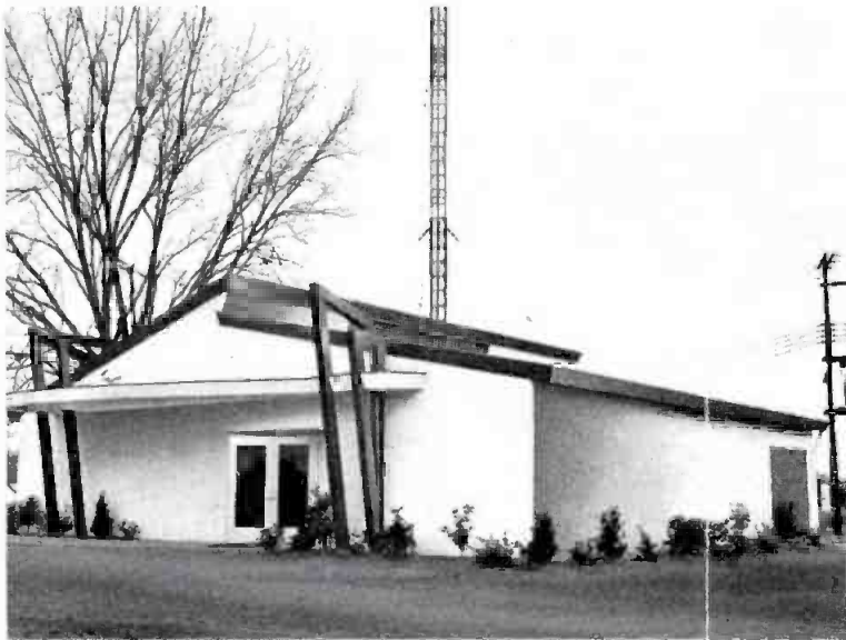
WKAB-TV, Mobile, Ala. G-E 12-kw transmitter in this modern building brings the first television service to the greater Gulf Coast area. WKAB-TV began operating with 12 kw August 5, 1953.
