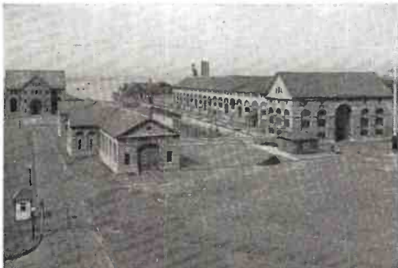
World's first major hydroelectric plant, built by the local electric company 58 years ago on the Niagara River above the falls and still operating.
