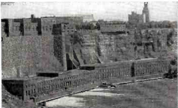
Another hydroelectric plant just below the falls . . . one of the more than 100 hydro plants operated by electric companies in New York State.
