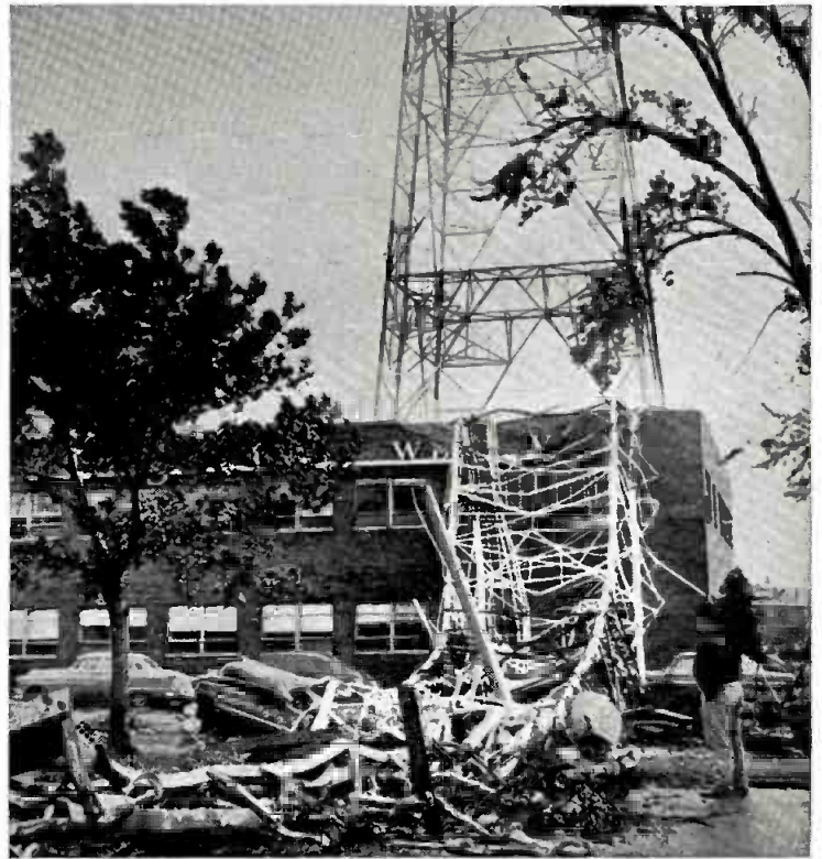
After the storm had done its damage.
