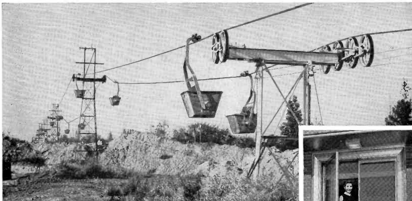
Swampland Bucket Brigade. This cable tramway stretches through 3½ miles of Georgia swamp, hauling clay to the plant of a brick company. The buckets are carried on an endless 30,000-foot length of USS Tiger Brand Wire Rope. In six years, the tramway has carried over a million tons of clay; it has reduced hauling costs by 66%.
