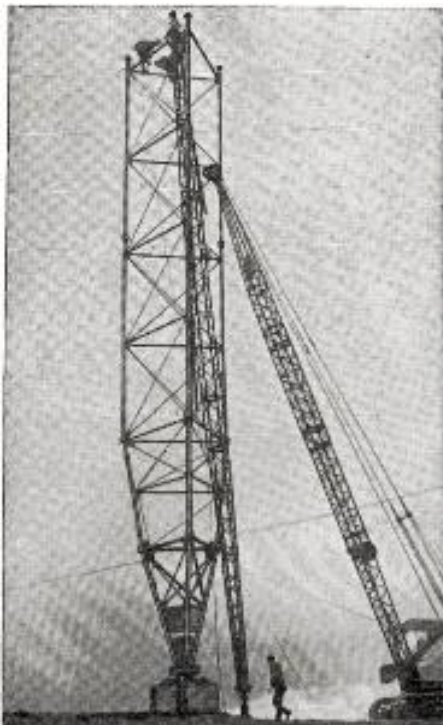
Construction close-up on new 1282-foot Truscon Triangular Guyed Tower for WTV in Cadillac, Mich.
