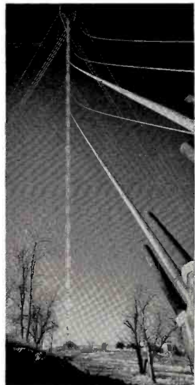
Tall Tale From Texas. This immense TV tower near Dallas is almost \frac{1}{3} of a mile high (1,521 feet to be exact). Naturally, they don't want it to fall down, so it is anchored with about five miles of USS Tiger Brand guy line. The guys range from 1\frac{3}{4} to 2 inches in diameter. They are anchored in concrete as far as 1,050 feet from the base of the tower.
