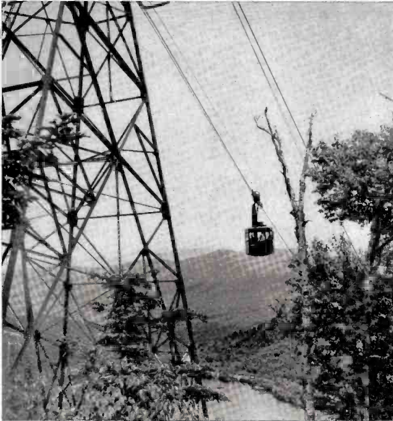
You'll Float Through The Air—For A Mile. This is a cable tramway for tourists that goes up Cannon Mountain at Franconia Notch in New Hampshire. The heavy wire ropes are well over a mile long, 1 7/8 inch in diameter and they weigh 28 tons apiece. The cable was made and installed by American Steel & Wire Division of United States Steel.
