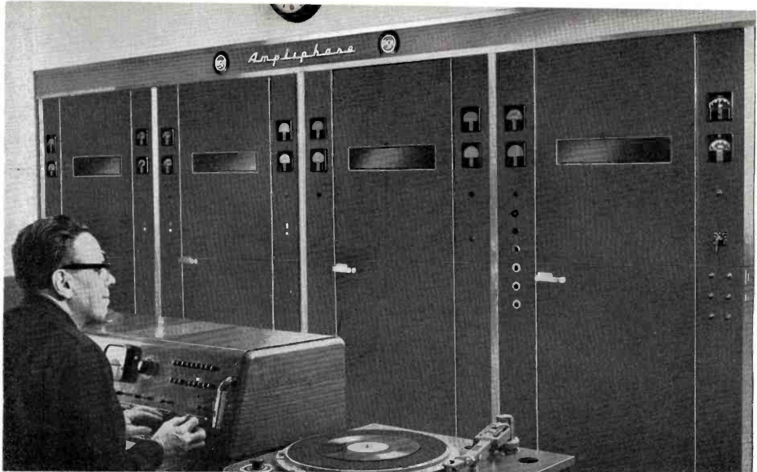
RCA Type BTA-50G transmitter at the WINS transmitter building in Lyndhurst, New Jersey, showing Al Jorgenson at Console.
