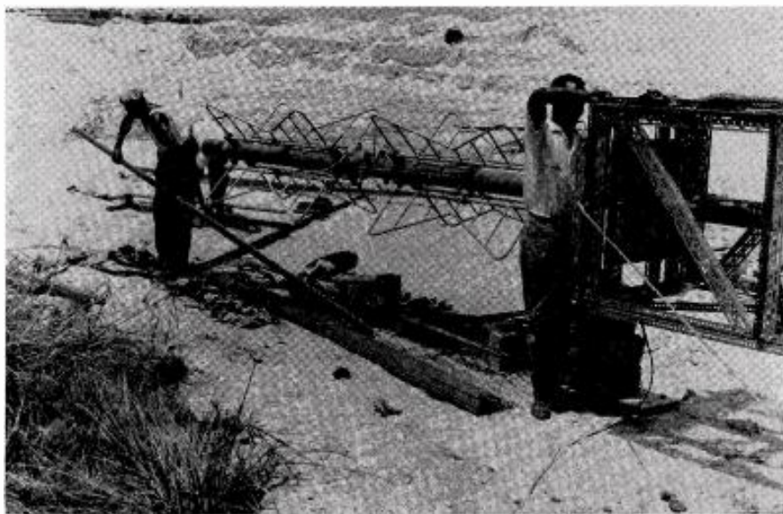
Natives in Lagos setting up antennas for the Nigerian Television Service.
