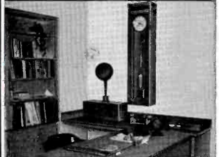
The gracefully-styled master Favag clock enhances the decor of Newman's private office, while acting as the nerve-center for the station's clock system.
