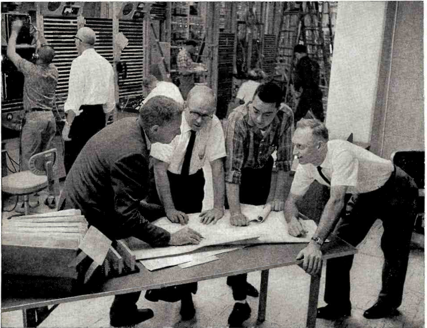
Teamwork. New switching equipment is installed at this Atlanta telephone central office of Southern Bell Telephone Company. Above, left to right, WE Engineer Van Van der Plaats, Nolen Ridgeway of WE Installation, Andy Anderson of Southern Bell and A. B. Johnson of A. T. & T. work out final details of the installation. For months before the cutover, Western Electric installers, systems equipment engineers and Southern Bell people worked side by side to complete these new facilities.
