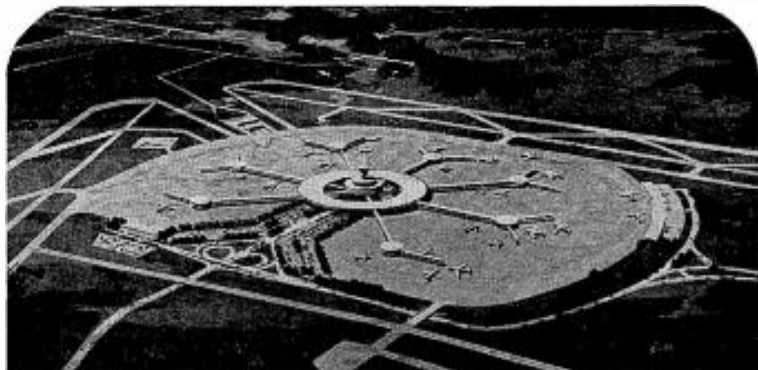
Houston's Intercontinental Airport, now under construction, will be completed in 1966, at a cost of approximately $150 million, and will be the only terminal in the Southwest capable of accommodating supersonic intercontinental jets.
