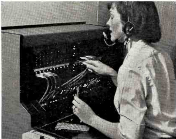
BLIND. Special "Seeing Aid" equipment has been designed so that blind operators can serve regular telephone switchboards. Its basic principle is a sensitive probe which causes a buzz in the operator's earphone when it passes over a lighted lamp. By moving probe up and down a central row of lamps, she learns what level the call is coming in on and which side. Then she uses probe to find proper hole and goes on to complete the call.
