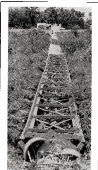
Tornado topples tower
